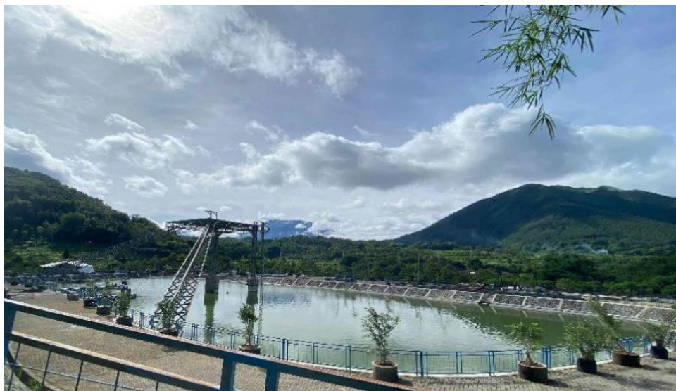
Figure 6.23 Application of Water Reservoir
