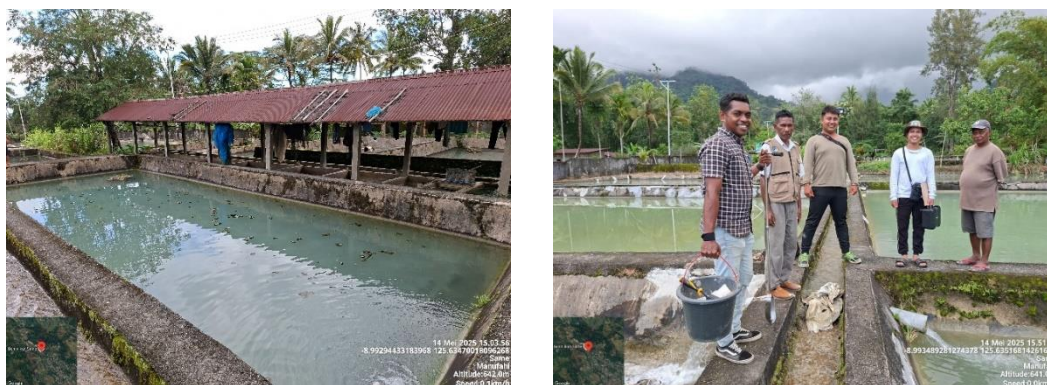
Figure 10.16 Freshwater Fish Farming Facility in Letefoho Village (Source: Research Documentation, 2025)
