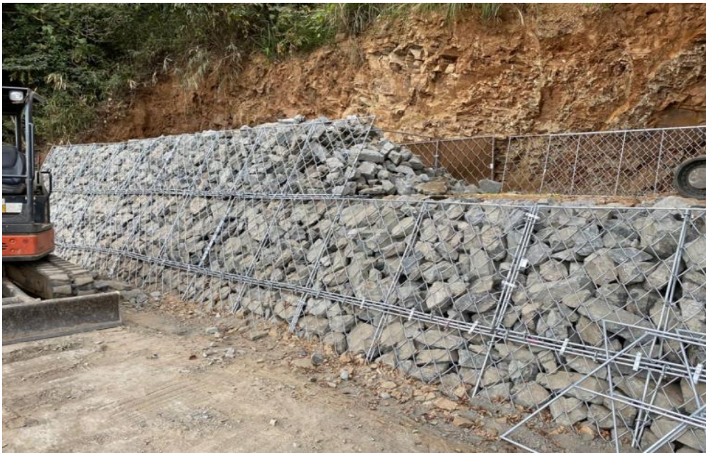
Figure 6.11 Gabion Check Dam
