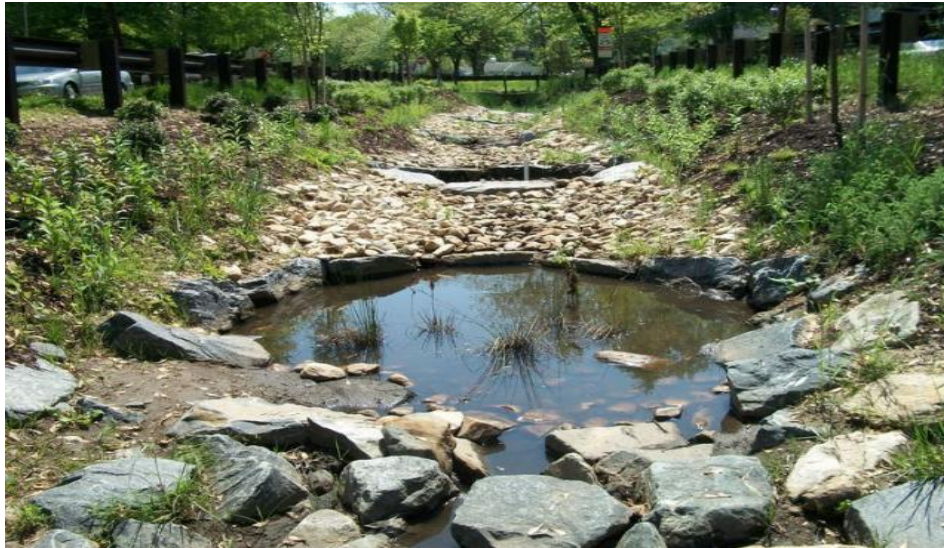
Figure 6.10 Loose Stone Check Dam
